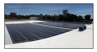
Novato and Sonoma based SolarCraft, recently completed the installation of a 113.2 kW solar power addition at Vineburg Storage in Vineburg, a community in Sonoma County, CA. The newly built facility will cut utility costs from the power grid while utilizing clean, renewable solar power to run their operation.
